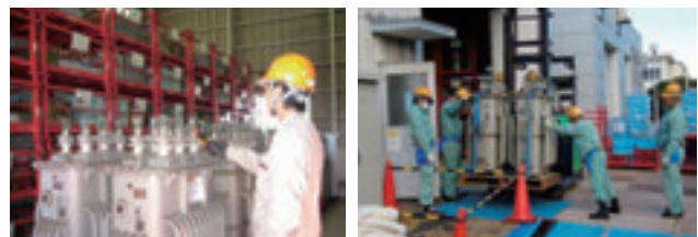
PCB-containing equipment being transported to Japan Environmental Safety Corp.
