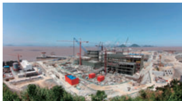
Construction of the Sanmen Nuclear Power Station in Zhejiang Province, China
