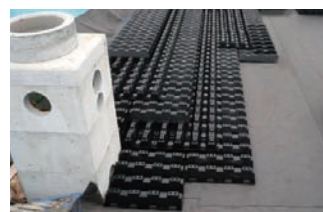
① System for draining rainwater into the ground
