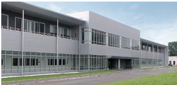
External appearance of the new building (Customer Support & Training Center)
